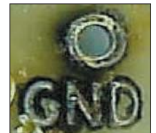
FIGURE 2: Sample of a corroded board.
